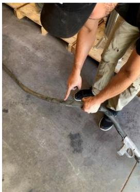
**Empty material from system** – If there is any remaining abrasive left within the system, empty the material into a bucket/container and store accordingly. With the Easy Blast 6, IBIX – Pro 3 and Pro 9, simply press open the flapper door, located on top of the system, with one hand. Once the flapper door is
